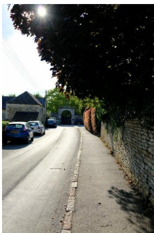
Picture 5 North Luffenham Pavement
